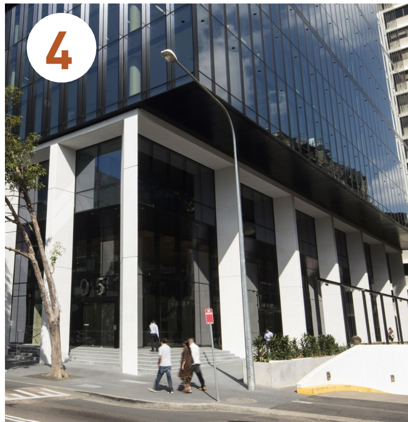
PRECAST CONCRETE VERTICAL AND HORIZONTAL RETAIL BLADES
